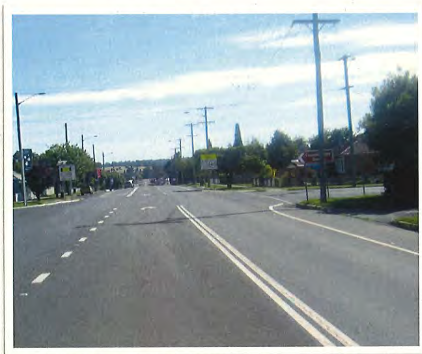
Plate 6. View or northerly approach – New England Highway
