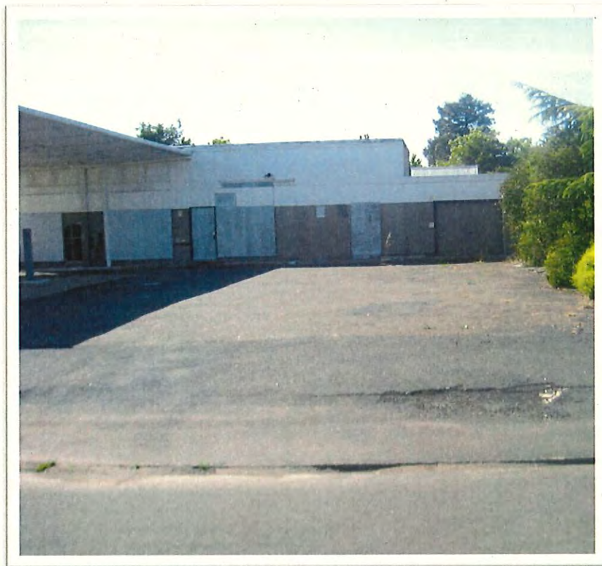
Plate 1 – View of existing building located on subject site.
