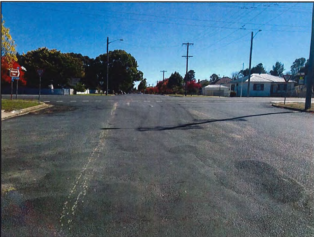
Photo 2 - Cross section of John Street looking west toward Bridge Street
